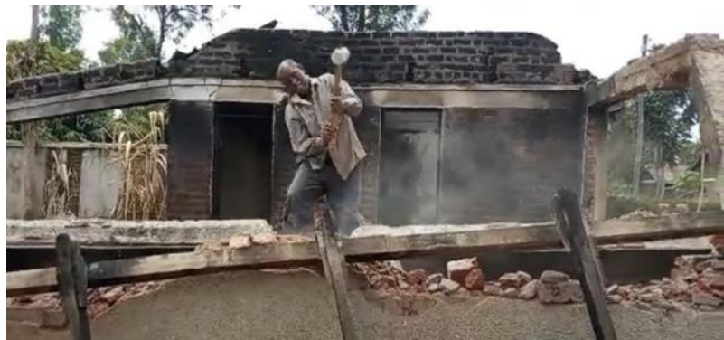
A KBC faculty member helping with the building demolition.
